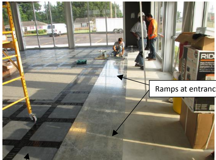
UniPanels starting from ramps (example of a chain store showroom)
